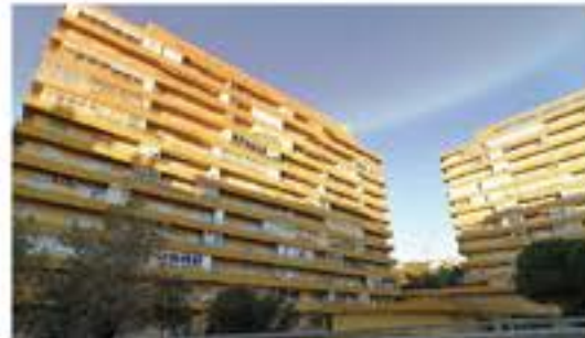
SPAIN-Staff Dormitory, Spain
