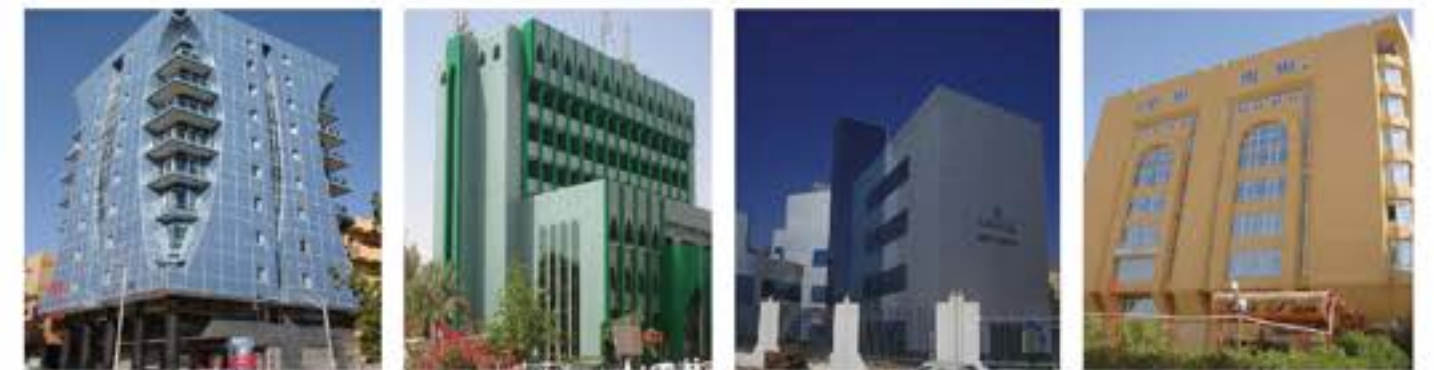
Sudan-Office Building, Sudan
